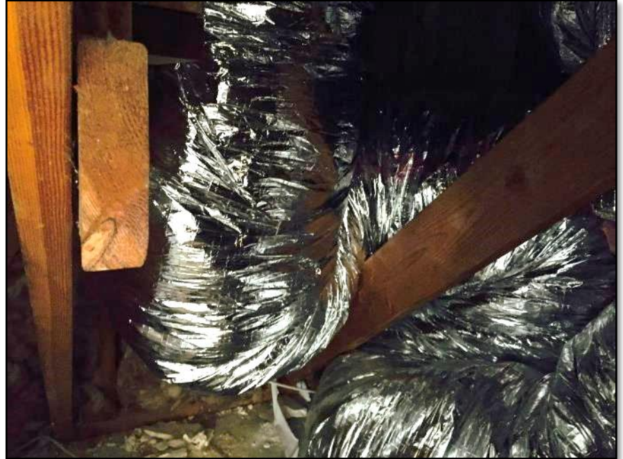
Poorly installed ducts
