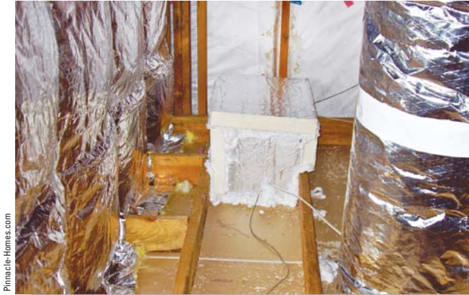
Fig. 9.11a Insulated, air-tight cover for a can light which penetrates the attic
