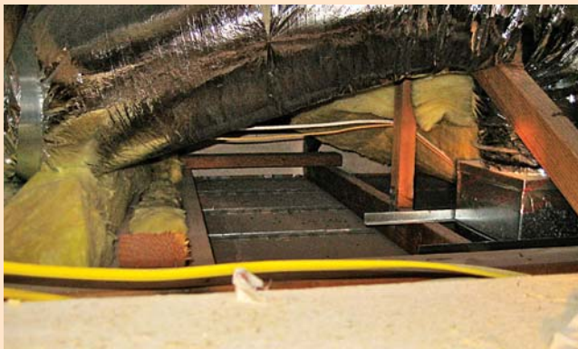
PAST PRACTICE... INSULATION IS "MISSING IN ACTION"
