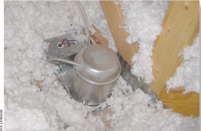
Fig. 2.9 Modern air-tight, IC-rated can light
