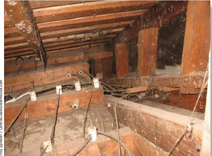
Fig. 6.4 Replace knob-and-tube wiring
