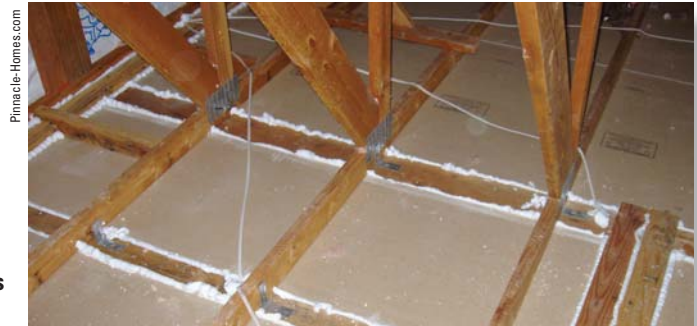
Fig. 3.7 Air sealing the assembly that separates the attic from the living space below.
