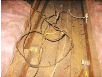
Fig. 3.9 Wiring deficiencies like this one are a fire hazard, and must be corrected before filling the attic with insulation
