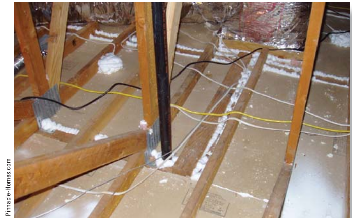
Fig. 9.13 Sealing the top plates of interior walls and the seams of ceiling gypsum board panels with spray foam Also note the foam-covered, air-sealed electrical box
