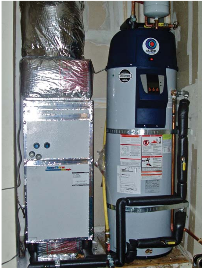
Fig. 8.4 Hydronic air handler, combined with a high-efficiency, sealed-combustion natural gas water heater
