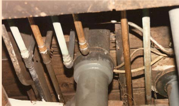
PLUMBING PENETRATIONS... PLUS LEAKY TONGUE & GROOVE FLOORING
