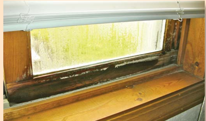
Fig. 10.2 Extensive frame damage - Consider replacement
