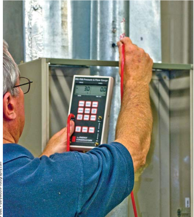
Fig. 5.11 Measuring exhaust vent draft suction Consult table 5.4 for minimum vent draft suction levels
