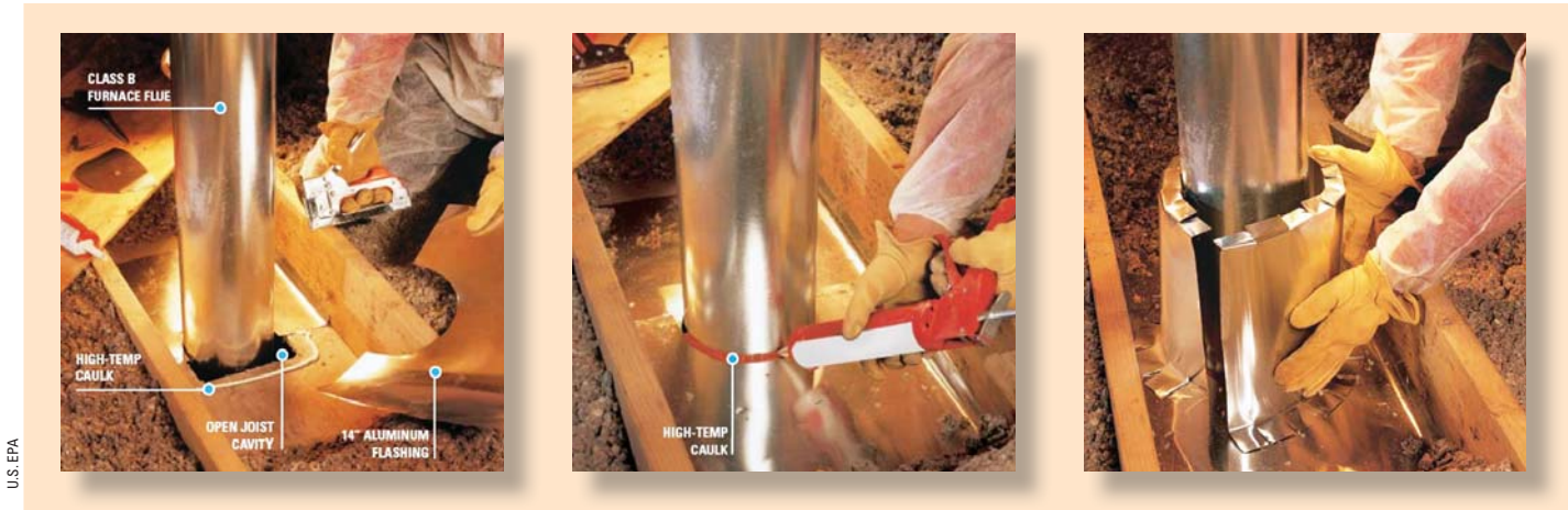
Fig. 9.9 Sealing a furnace flue which penetrates the attic
