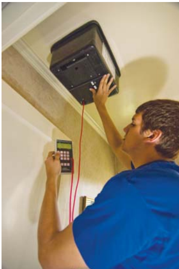
Fig. 3.11 Measuring and setting air flows to each room
