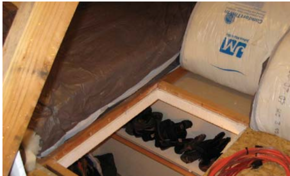
Fig. 9.6 Attic access hatchway
