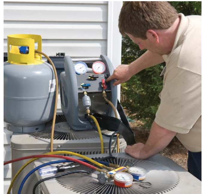
Fig. 3.12 Measuring and adjusting the refrigerant charge of the AC system, based on its operating load
