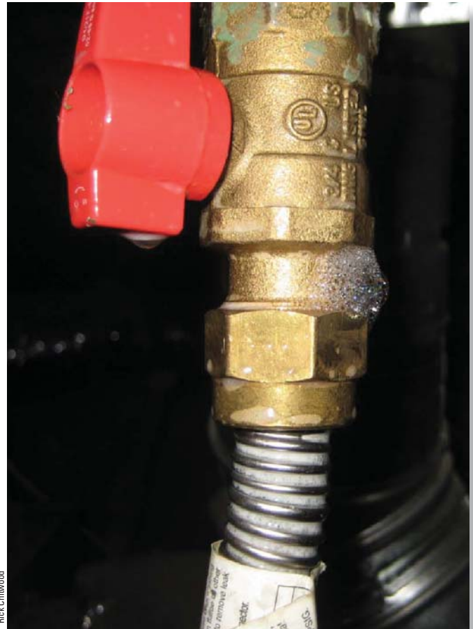
Fig. 5.14 Detergent solution - Visual gas leak detection
