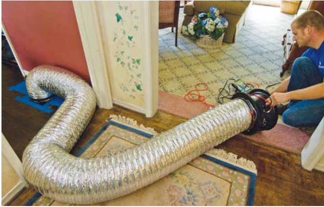
Fig. 3.10 - Measuring duct tightness
