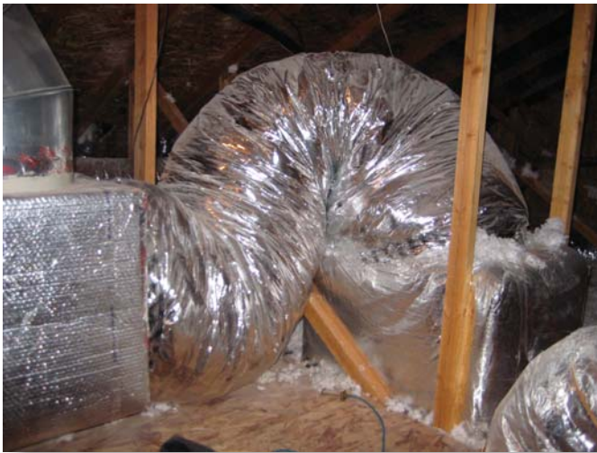
Fig. 2.6 Duct design and installation affects energy consumption more than the SEER rating of the AC unit
